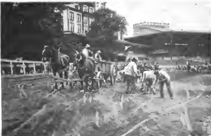
REPAIRING THE MUCH CUT-UP TRACK DURING INTERMISSION.
